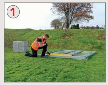
The Adman installation team will level the base frame and assemble the Multigrow Greenhouse.
