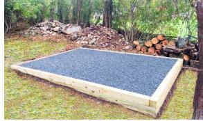
**N.B.** Air must be allowed to flow above and below the Timber Floor. Do not cover the floor internally with lino or carpet.
