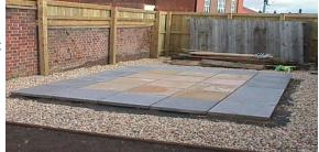
N.B. Air must be allowed to flow above and below the Timber Floor. Do not cover the floor internally with lino or carpet.
