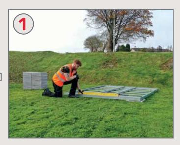
The Adman installation team will level the base frame and assemble the Multigrow Greenhouse.
